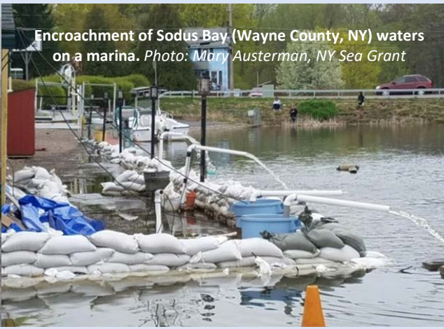
Inundation of Greene Point Road (Oswego County, NY). Photo: Cathy Goodnough
